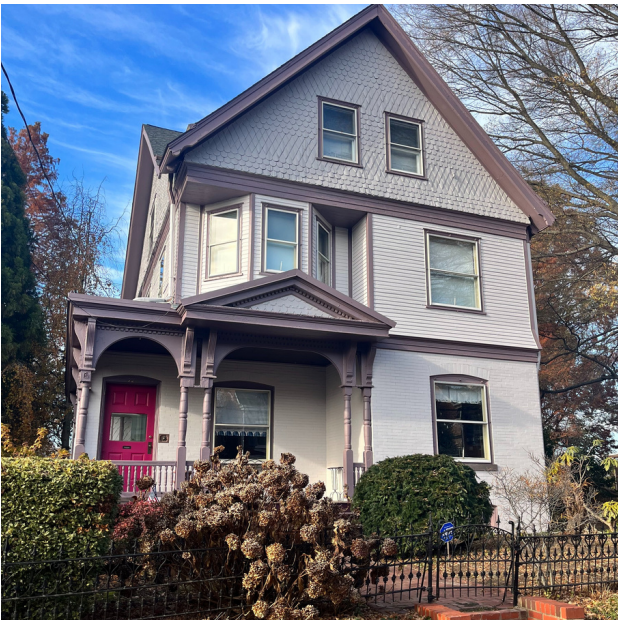
Small Project rehabilitation located in the Historic District of New Castle
