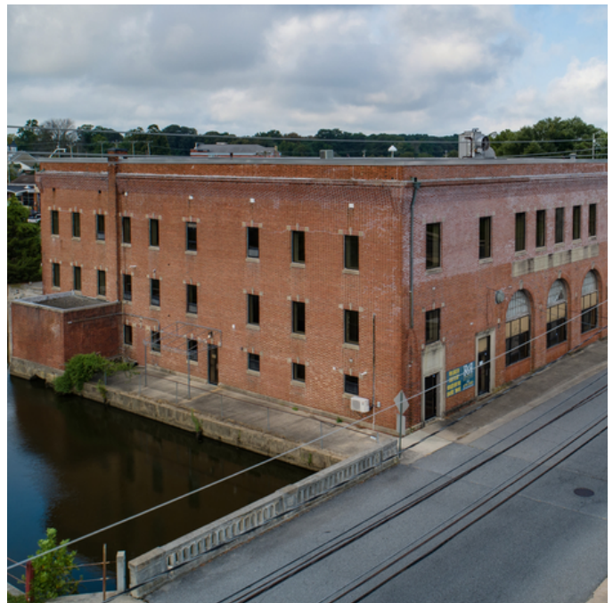
Old Carlise Firehouse in Milford
