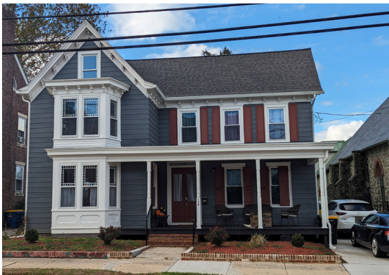
Rehabilitation of existing residential home
