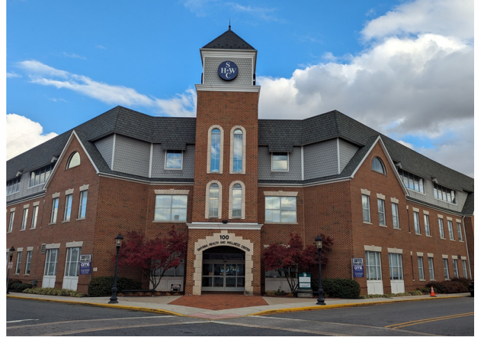
Rehabilitation of existing building improved to function as a modern orthodontic office.
