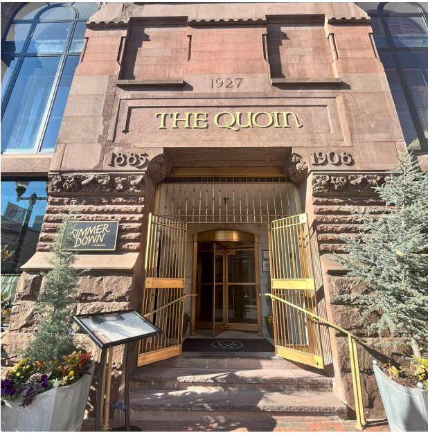
Large Project rehabilitation in Wilmington
