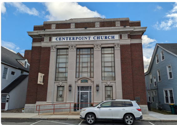
Rehabilitation of existing bank building
